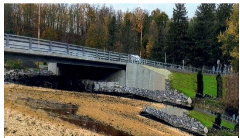
bridge over Oriskany Creek - 2016
