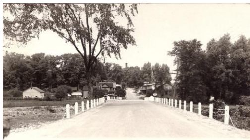
bridge over Oriskany Creek - 1936
